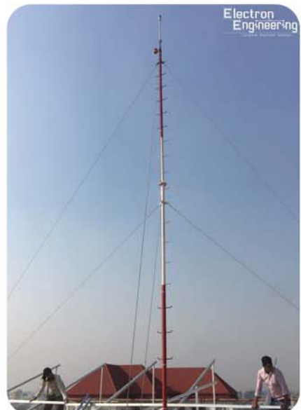
Exim Bank Head office Gulshan-1
